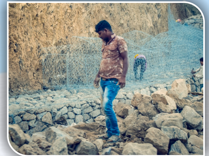
“Slope stability work of Himalayan Mountainous terrain using Geo Grid”
